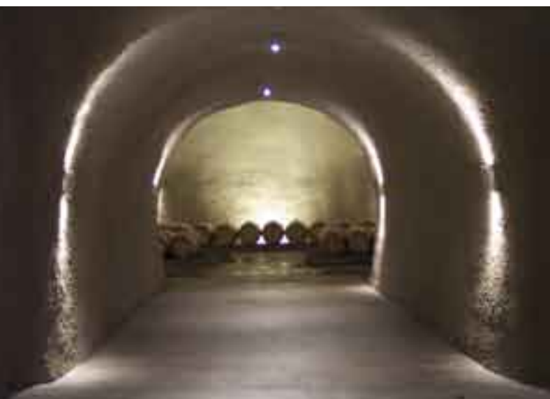
Access portals lead to the main chamber.
