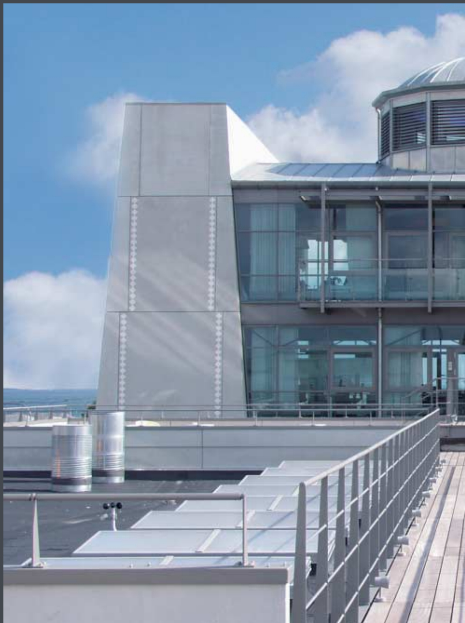
The two AALBORG WHITE® based concrete towers frame the lightweight glass sections.
