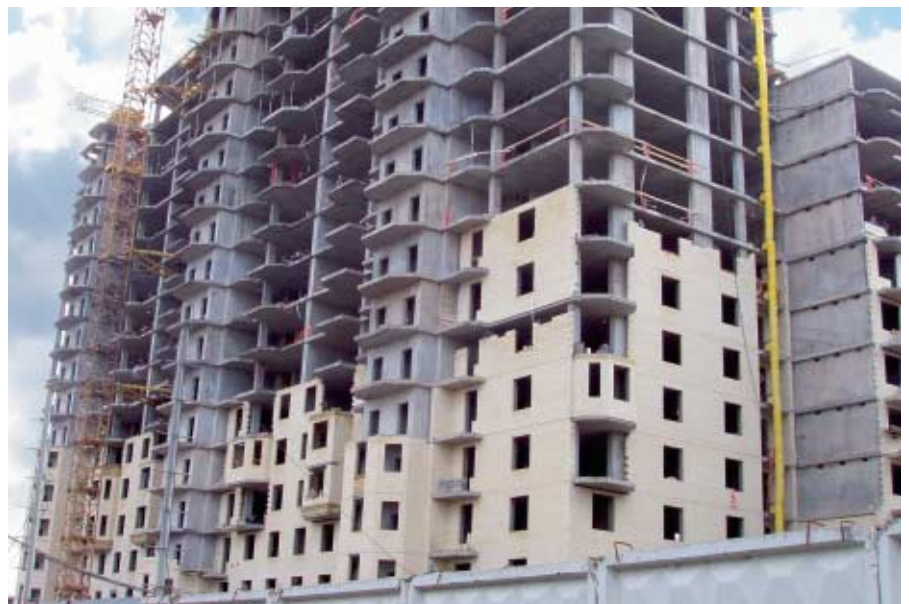
A project currently being implemented is the construction of fifteen 22-storey buildings in white brick and concrete on a site close to Moscow State University.
